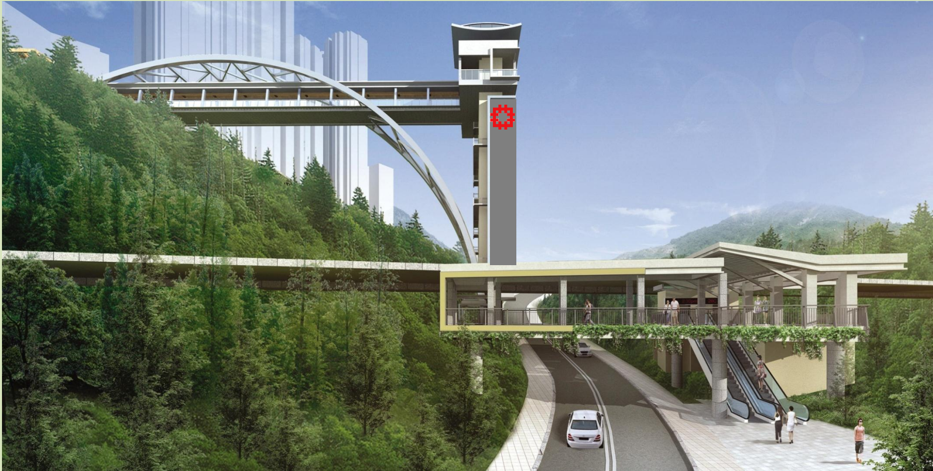
Footbridges at Shui Chuen Au Street
