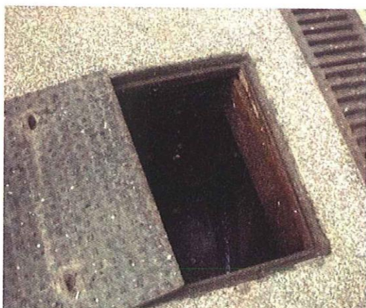
Manhole condition after high water pressure jetting cleaning.
