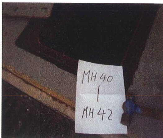
High water pressure jetting cleaning in manhole no. MH40 to MH 42.
