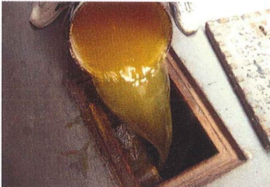
Dye Test for manhole near flat 103 to flat 106 at East
