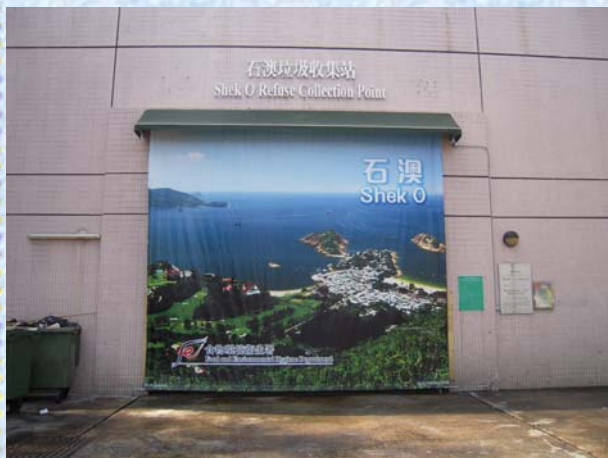
Shek O Refuse Collection Point
