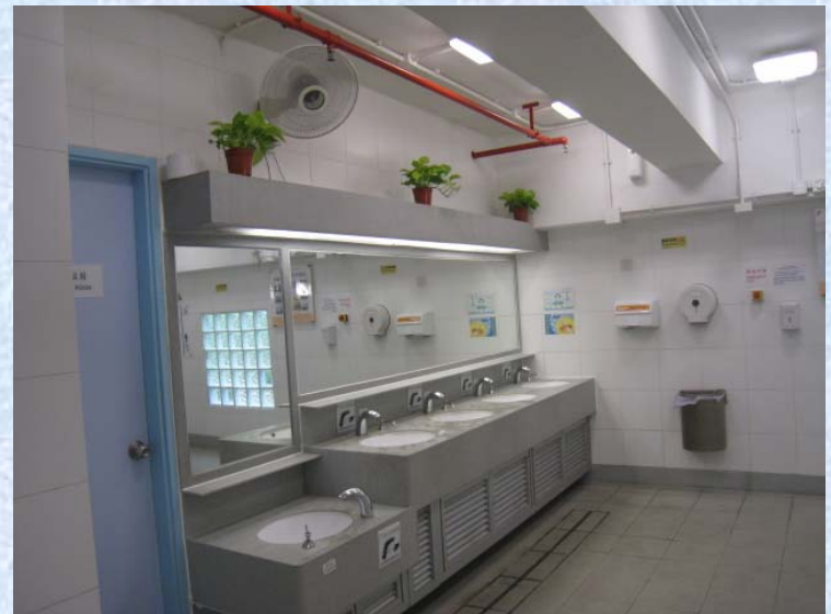
Internal Setting of Public Toilet in Apleichau Municipal Services Building
