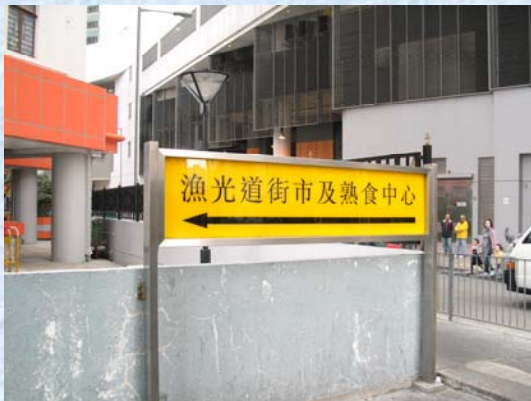
改善工程前 Before beautification works
