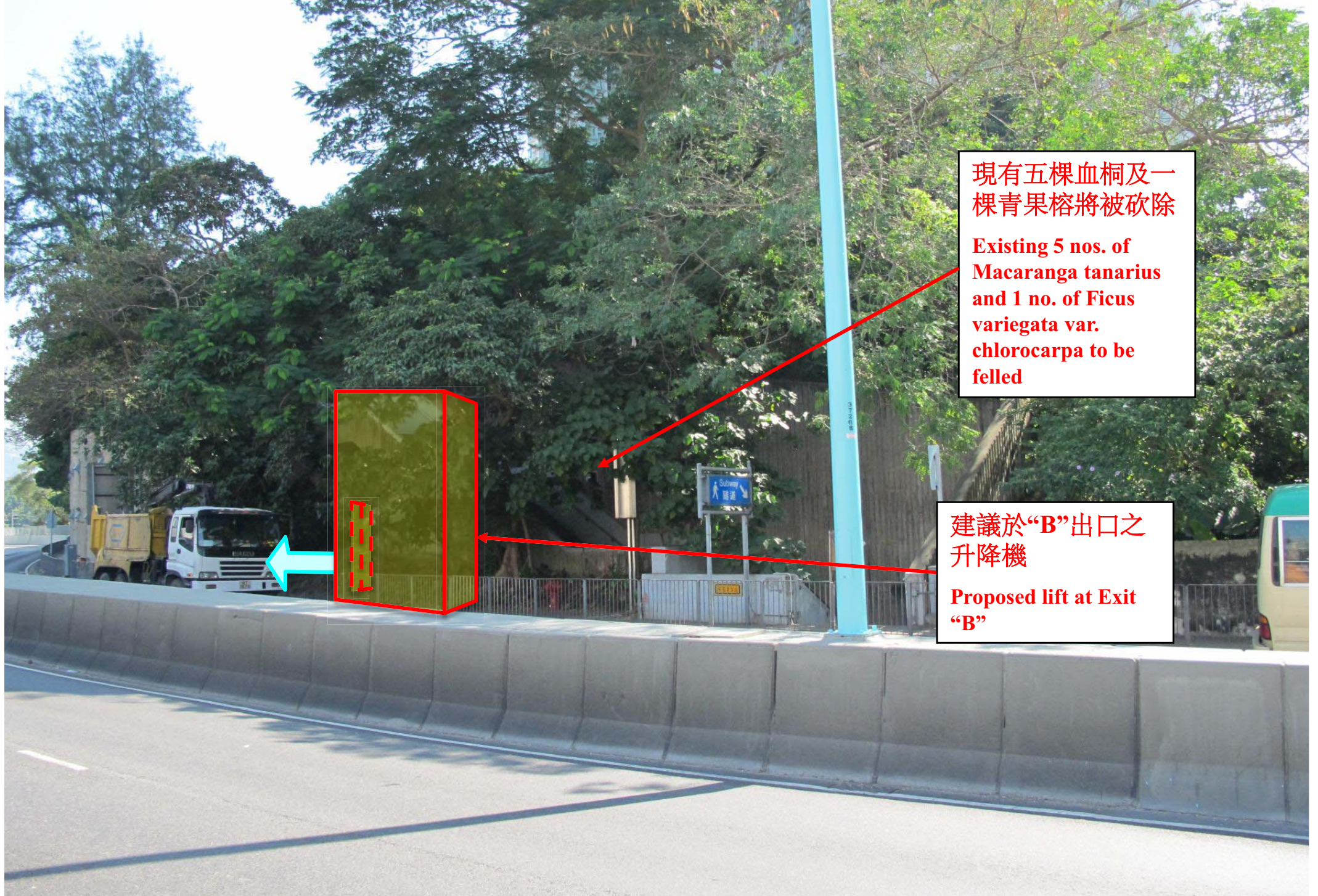
附圖 6 (行人隧道編號 HS13 及 HS13A - 建議於“B”出口之升降機) Figure 6 (Proposed lift at Exit “B” of existing subway nos. HS13 and HS13A)
