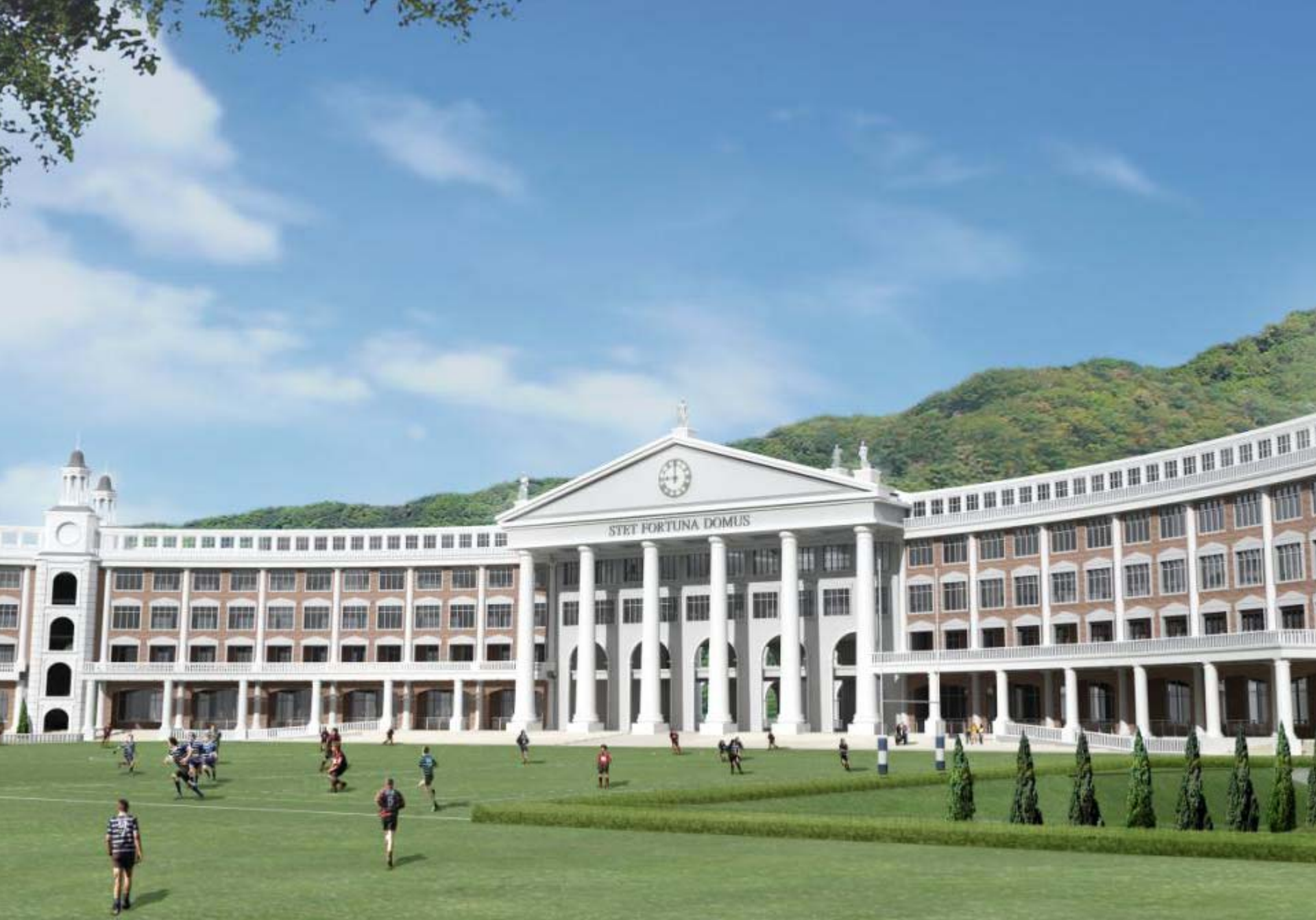
主入口近觀 Close up view of Main Entrance
