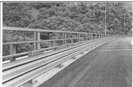
現有橋樑護欄加裝附加柱、橫杆及三波板防撞欄 UPGRADING OF EXISTING 3-RAIL STEEL PARAPET WITH THREE BEAM
