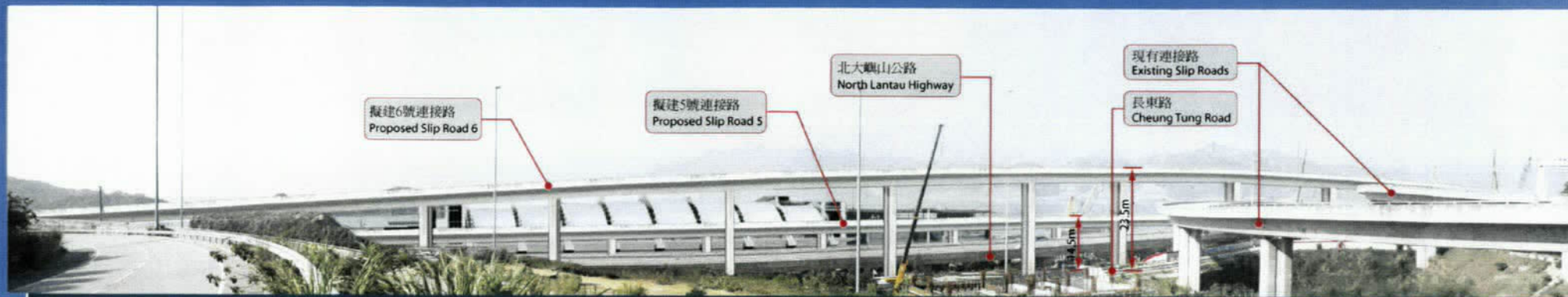
View North from Existing Link Road 1
