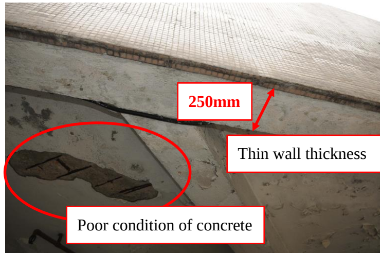
Photo 2.3 – Existing condition of nearby building
