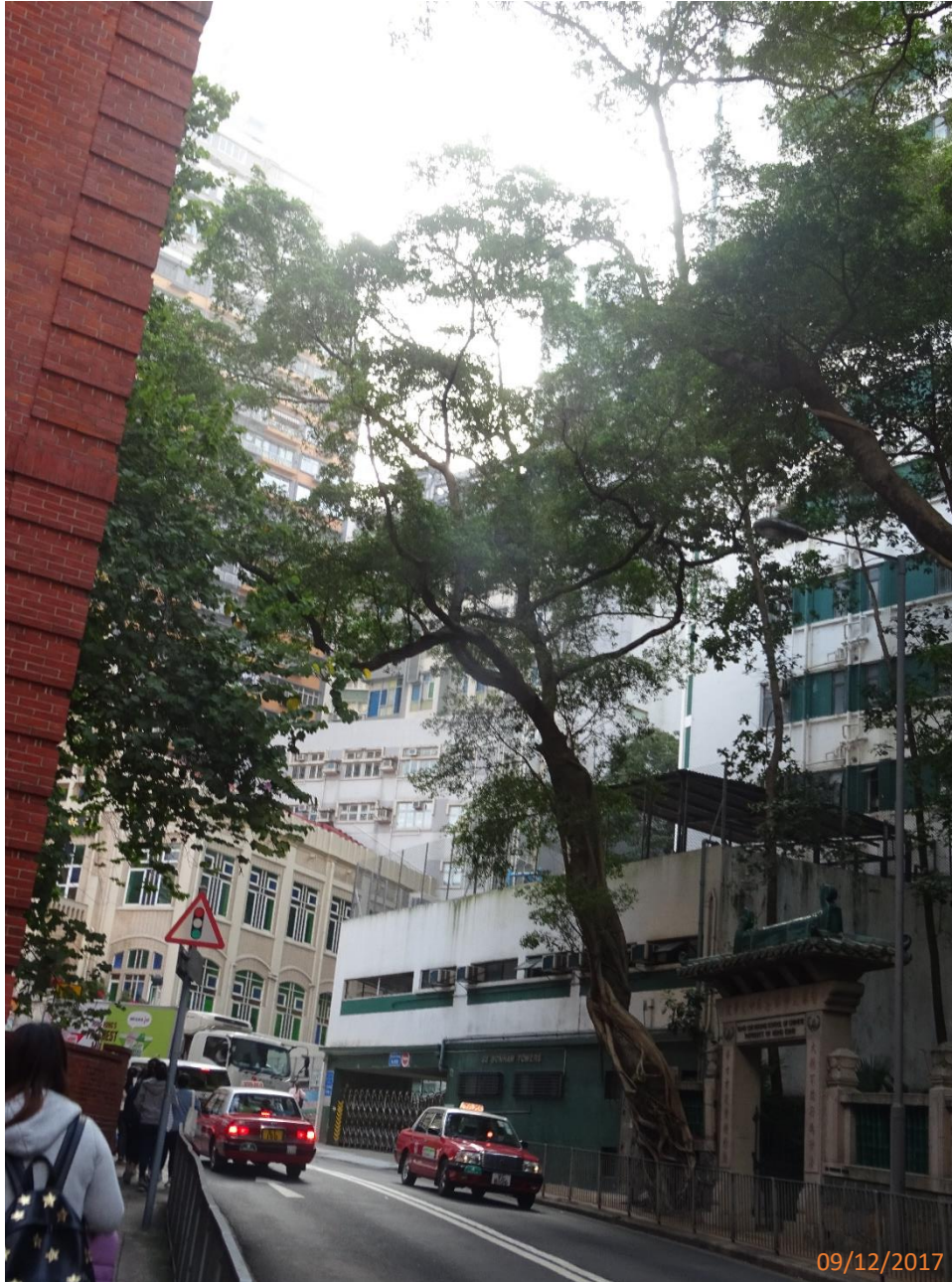
Overview of T1: Leaning at about 30 degree towards the Bonham Road
