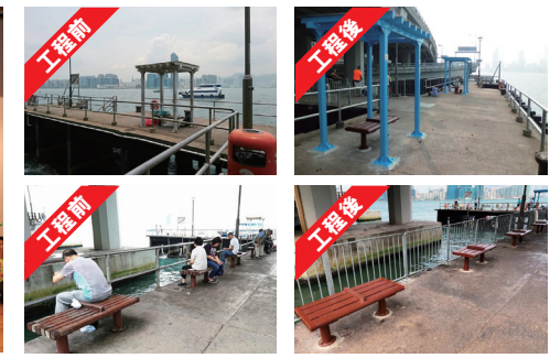
▲北角糖水道碼頭重建避雨上蓋及座椅
