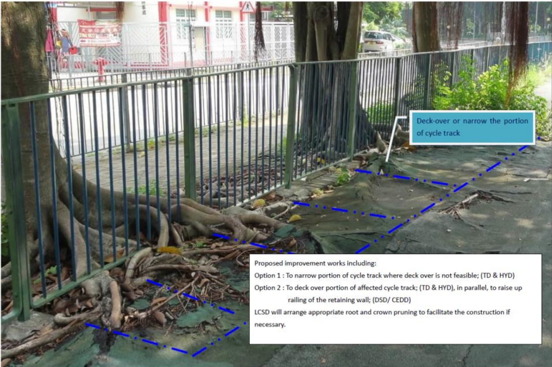
(II) Portion of pavement with protruding tree roots from roadside trees planted on the pavement (about 58 nos. of trees)
