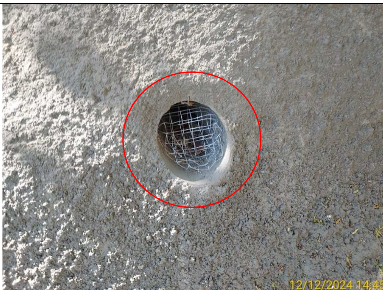
Photo 12: After - Installed wire mesh to prevent drain holes from becoming rat holes.
