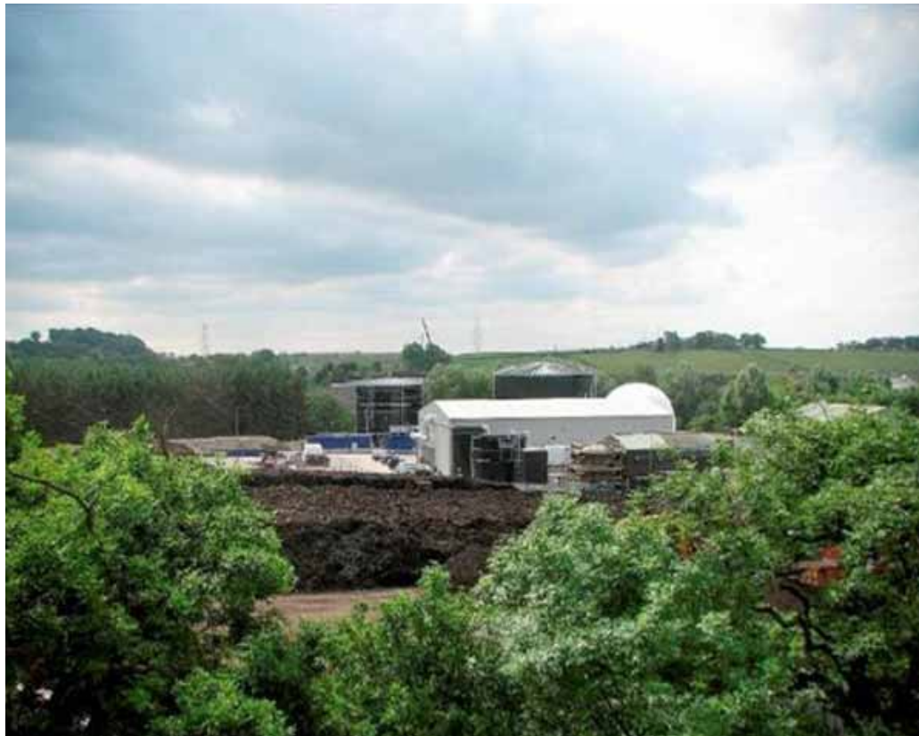
圖片資料: Deerdykes Composting and Organics Recycling Facility (Mott MacDonald UK)
