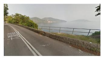
A narrow section of Tai Tam Road (Red Hill to Stanley) adjacent to a 20m high sea cliff. The stone wall does not have the capability to resist impact by buses and coaches at general speeds.
