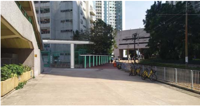
WCWP International Limited 15013-009-TM-DMW-221- Construction of Covered Walkway in Tuen Mun District (Phase 2)- Yuet Wu Section
