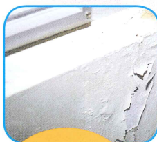
牆身/窗邊滲漏 Seepage from the walls and window sides
