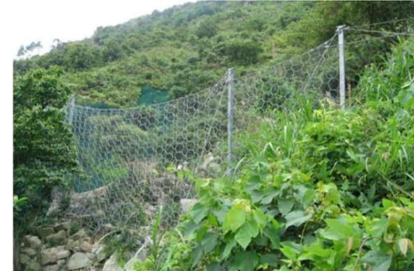
Photo of Debris-resisting Flexible Barrier
