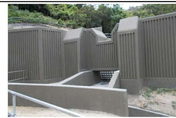
Photo of Debris-resisting Rigid Barrier
